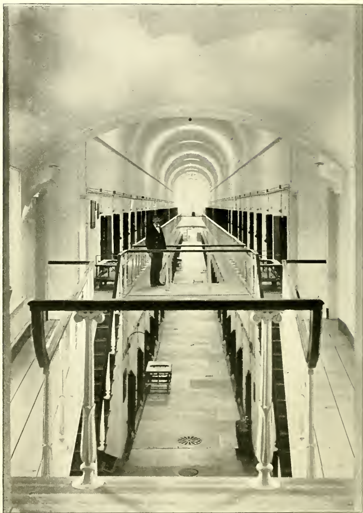
Seventh Block (two stories)—365 ft. long, 10 ft. wide, 38 ft. high—136 Rooms, 16x7 ft. 6 in., 11 ft. high—Eastern State Penitentiary.
